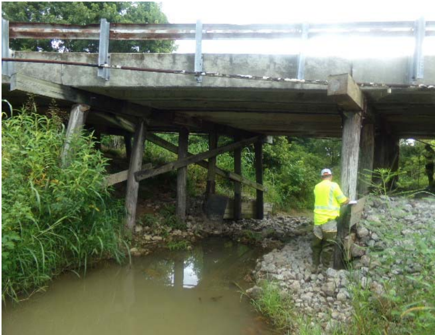
WASH BENT # 2 PILE "D" UNDER CASING
