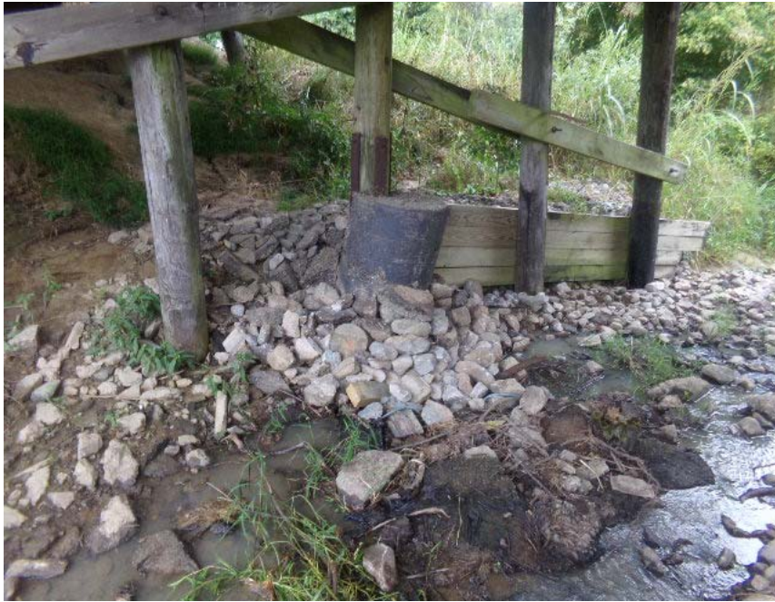
BENT # 2 PILE "C" RIP RAP
